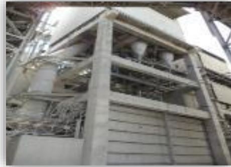
2007 : Line-1 upgradation with conversion into Close circuit
